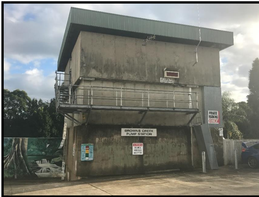
Figure 2: Brown Street Pumping Station
