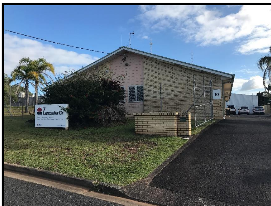
Figure 9: SES Region Headquarters Richmond Tweed
