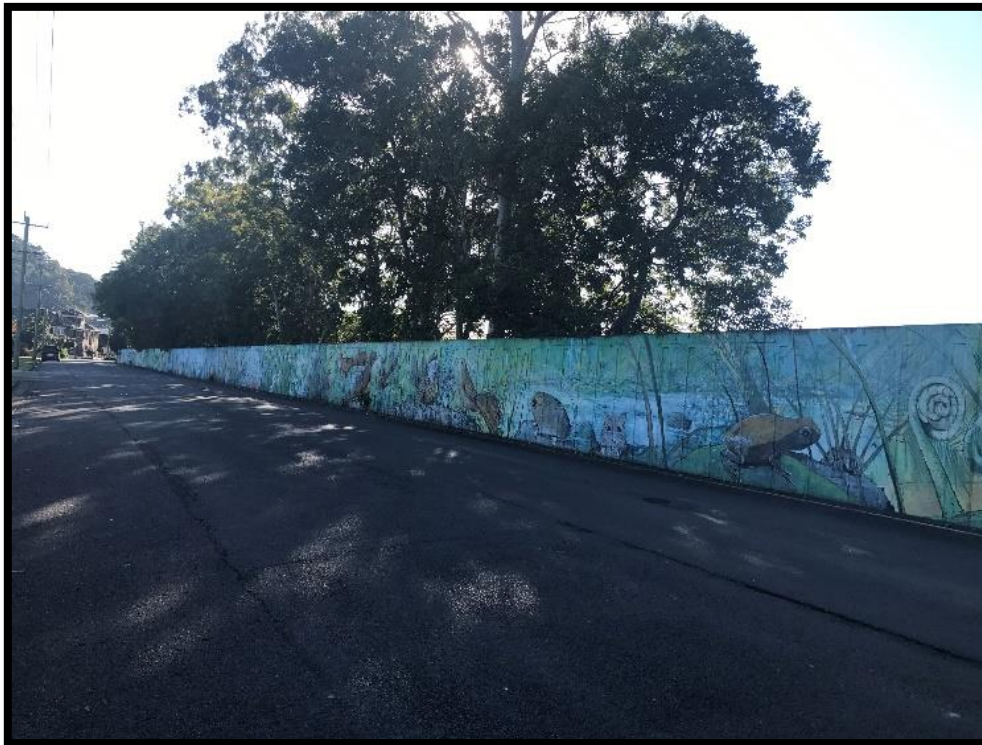
Figure 3: Commercial Road Levee wall (Murwillumbah)
